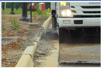
BULKY DEBRIS REMOVAL AND CONSTRUCTION SITE CLEANUP
