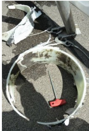
Step 2: Remove the liner cutout
