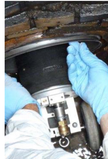
Step 4: Install using packer
