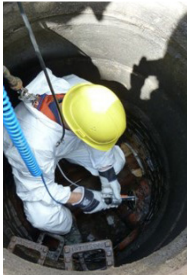
Step 1: Cut out the liner end
